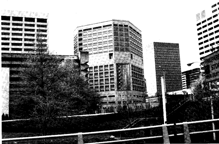
The towering Justice Center Jail in Portland held the suspects until their trials.
